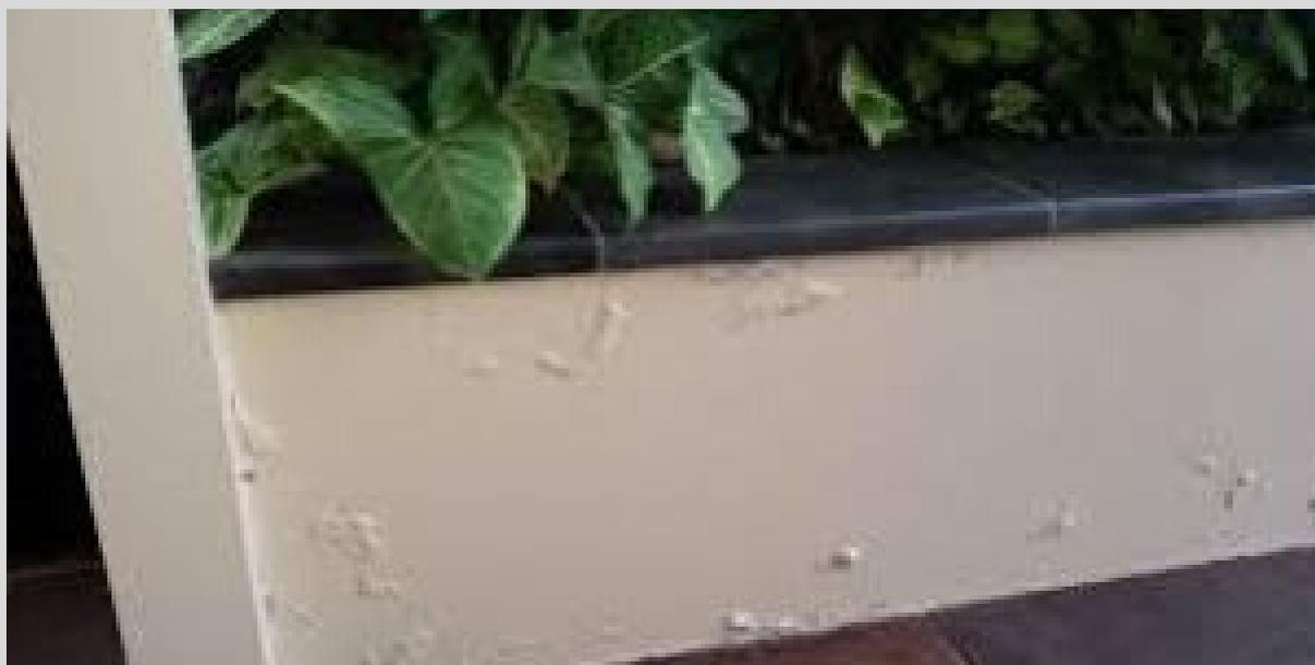
A common problem with walls and floors that are effectively underground or have earth back-fill against the external surface is that they range from being always damp to water seeping through them.
